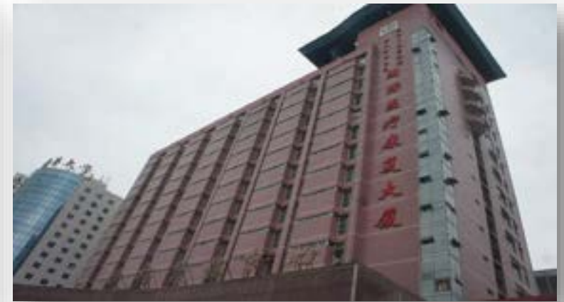
Hospital de Tian Jin
