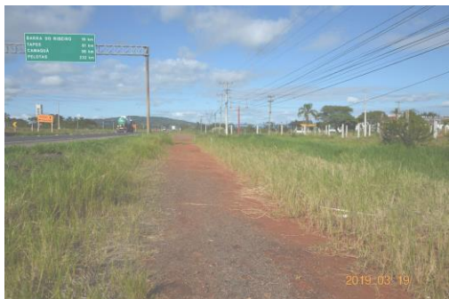
Figura 60- A jusante do BTTC 1,0
