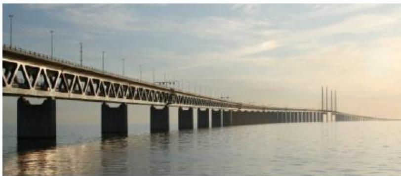
*The Øresund Bridge connecting Sweden and Denmark was constructed with steel containing .022% niobium. This reduced the weight of the bridge by 15Kt and saved US\$25 million in construction costs.*
