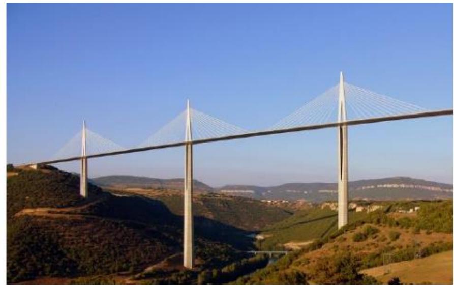
*The Millau Valley bridge in southern France was built using steel with 0.025% niobium. This reduced the weight of the steel and concrete by 60%*
